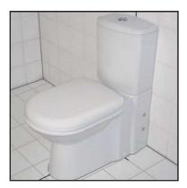
17 Check the final balance with a water gauge. Test the wc pan for a possible leakage. Silicone based pastes may be applied on the joining edges of the ceramic and finished wall for a better tightness and aesthetic view.
