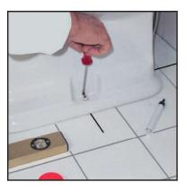
5 Place the bidet to its final position and fix it by using its original assembly kit.
