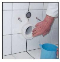
Prepare the waste outlet. Slide the eccentrical trap adapter in.
