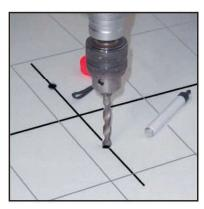
$\boldsymbol{6}$   $\,$  Drill the marked points with suitable drill bits and insert the raw plugs.
