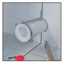
2 Fix the straight pipe to the ring, join it with the waste water outlet on the wall. Fix the ring to the wall.
