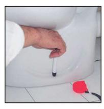
5 Bring the wc pan temporarly to assembly position. Mark the holes on both sides on to the finished floor.
