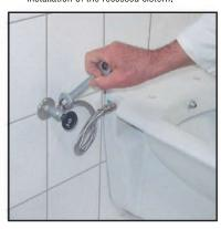
4 Connect hidden lustration system with connection adapter for WC pan.
