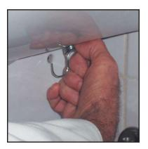
The main body of the assembly kit is fixed to washbasin assembly bolt, with the help of nuts, as shown on the above.
