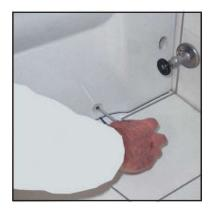
10 Slide assembly screws trough plastic bushes and screw to main mounts at both sides of the bidet.
