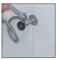
$6 \;\;$  Finish with the connections between interval taps and the bidet tap.
