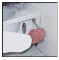
3 Push the bidet forward to assembly position. Slide the syphon trough the waste water outlet. Fix the assembly nuts of the bidet.
