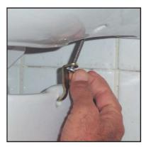
After fixing both hooks, begin to screw the bolt by hand. See the semi pedestal starts to rise slowly and get closer to washbasin
