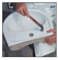
The central tap holes are left open during the mass production. For recessed tap systems; the closed holes at left and right sides must be open with a sharp pointed hammer with patience, from the top.
