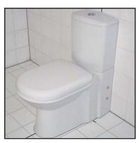
Check the final balance with a water gauge. Test the wc pan for a possible leakage. Silicone based pastes may be applied on the joining edges of the ceramic and finished wall for a better tightness and aesthetic view.
