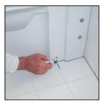
5 Use the projection of the WC pan and assembly holes at sides as template and trace contour lines on the floor.
