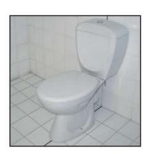
9 Test the wc pan for a possible leakage. Silicone based pastes may be applied on the joining edges of the ceramic and finished wall for a better tightness and aesthetic view.
