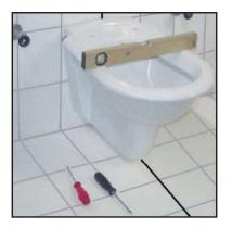
3 Place the wc pans to final assembly position and fix it by tighten the nuts trough the assembly bolts of the recessed cistern.
