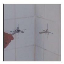
Prepare the waste water outlet and clean water inlets as given on product specification page. Temporarily place the basin, that its front will be at 800 mm. above the finished floor. Mark the assembly points on the wall. Drill the points with suitable bits, insert the plugs. Then screw the assembly bolts trough the raw plugs.
