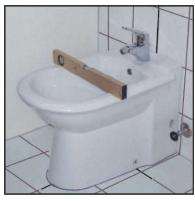
Place the bidet temporarly to assembly position. Use the assembly holes as reference points and mark the projections on the finished floor.
