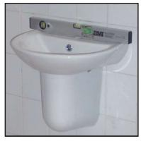
12 Check the final balance with a water gauge. Test the tap and look for a possible leakage. Silicone based pastes may be applied on the joining edges of the ceramic and finished wall for a better tightness and aesthetic view.
