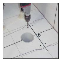
10 Overlap the strip's "+" sign with the intersection of axis on the floor. Now, mark the holes of the main mounts on the strip. Drill them.
