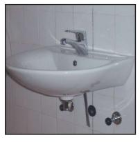
Drill the holes with suitable bits, insert raw plugs. Install the interval taps for clean water and washbasin tap. Slide the plastic bushes and washers, screw the nuts.
