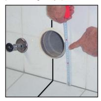
1 The centre of waste water outlet on the wall must be set to 170 mm. above the finished floor and the same level with the finished wall
