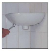
Mount the tap and syphon on the corner basin. Place the basin on the assembly bolts, insert the plastic bushes and fix the bolts with nuts.
