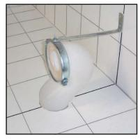
3 Fix the special "S" pipe to the ring, join the "S" pipe with the waste water pipe on the floor. Fix the ring to the wall with "S" pipe on it
