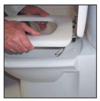
14 Each WC pan has its own seat cover, Thus, place the seat cover with its hinges on it, by sliding the screws trough installation holes on the pan.
