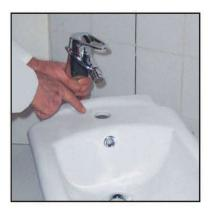
1 Set the gap between interval tap inlets to 400 mm. symmetrically regarding the centre as basis. Install the tap.
