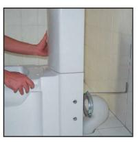
5 Install the cistern on the WC pan and place it temporarly to assembly position.
