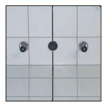
The waste water centre (Ø50 mm) is prepared at 125 mm above the finished floor. Set the gap between interval tap inlets to 400 mm. symmetrically regarding the centre as basis.
