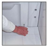
14 Place the wc pan to final assembly position. Slide assembly screws trough plastic bushes and screw to main mounts at both sides of the WC pan.
