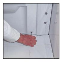
Place the wc pan to final assembly position. Slide assembly screws trough plastic bushes and screw to main mounts at both sides of the WC pan.
