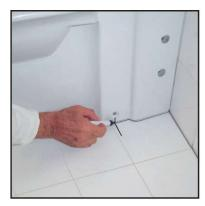
6 Use the projection of the WC pan and assembly holes at sides as template and trace contour lines on the floor.
