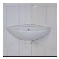
After fixing the washbasin, make the connections between interval taps and basin tap. Silicone based pastes may be applied on the joining edges of the ceramic and finished wall for a better tightness and aesthetic view.
