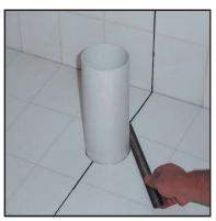
The waste water pipe on the floor is left at an extended height to set it up later. At the beginning of the installation, the extension will be cut off as shown.
