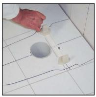
Join the markings at the 6th figure horizontally. Intersect it also with the vertical axis drawn before.
