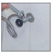
4 Prepare and finish the connections between bidet tap and interval taps.
