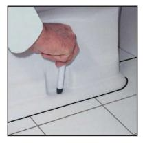
3 Keep this distance and mark the projection of the bidet and assembly holes on the finished floor.
