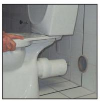
4 Slide the eccentrical trap adapter to the outlet of the wc pan. Calculate the gap, which is needed for extension for the waste piping.
