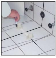
Join the markings at the 4th figure horizontally. Intersect it also with the vertical axis drawn before. Overlap the strip's "+" sign with the intersection of axis on the floor. Now, mark the holes of the main mounts on the strip.
