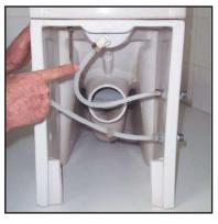
$13 \ \ {\small \hbox{Check all connections and hoses against} \atop \hbox{leakage}.}$
