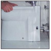
Push the bidet forward to assembly position. Slide the syphon trough the waste water outlet.
